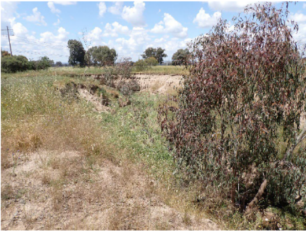
Figure 47 – SU9, significant erosion in creek line; view east from north bank.
