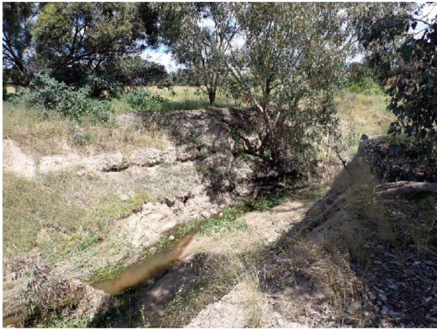
Figure 48 – SU9, significant erosion in creek line; view south-west from north bank.
