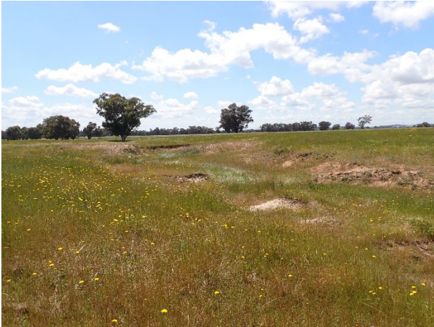
Figure 23 – SU3, Eroded creek banks, view west.
